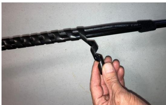
32. It may help to bundle the excess wrap with an elastic band so you can more easily move it round and round the cable and wands without getting in a tangle.
