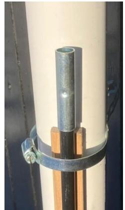
**Fixing to an existing circular post.** The first wand could be fixed to a circular post with two long worm-drive hose clips such as are available from Amazon or [B&Q](#) etc.
