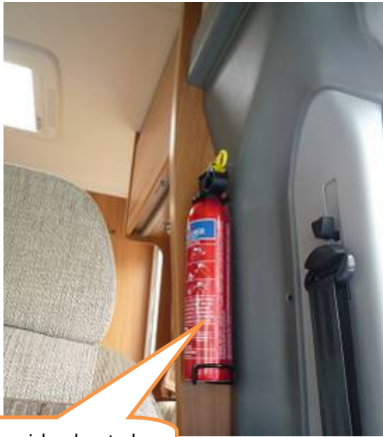
Fire extinguisher located behind passenger front seat
